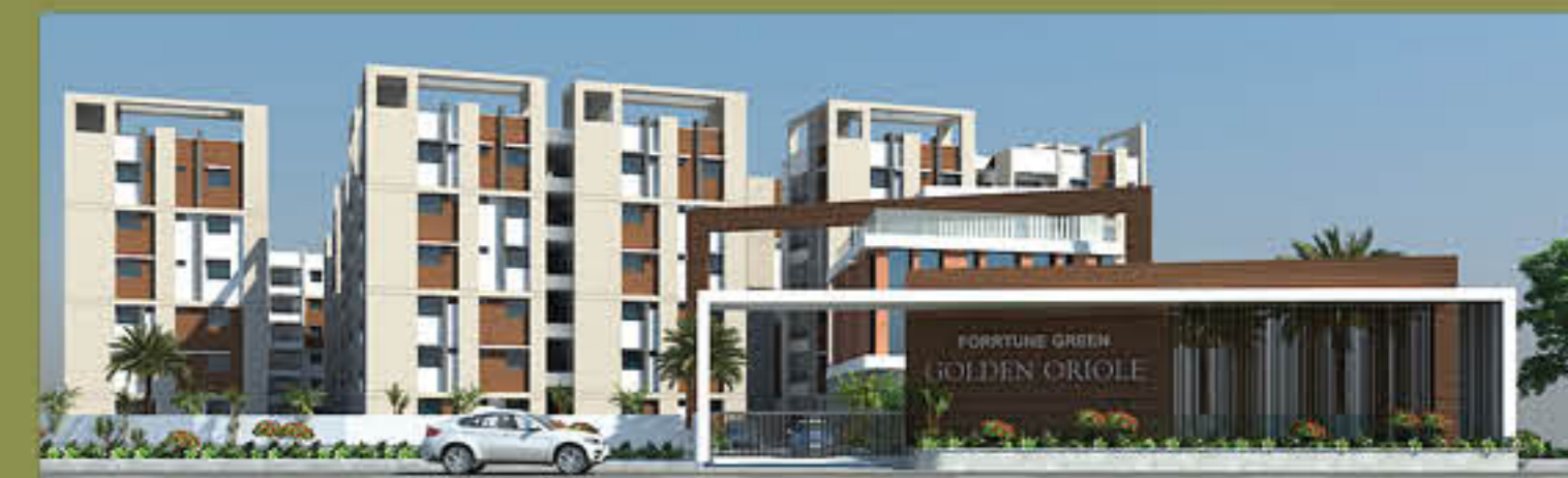
GOLDEN ORIOLE @ Narsingi, Puppalaguda, Pipeline Main Road.
